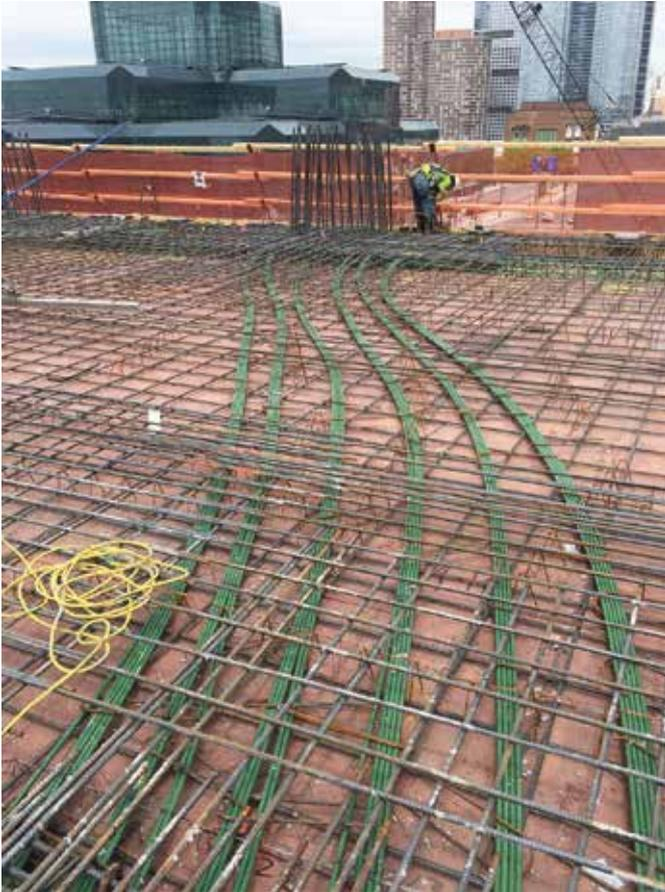
Fig. 4: Layout of post-tensioning and nonprestressed reinforcement
