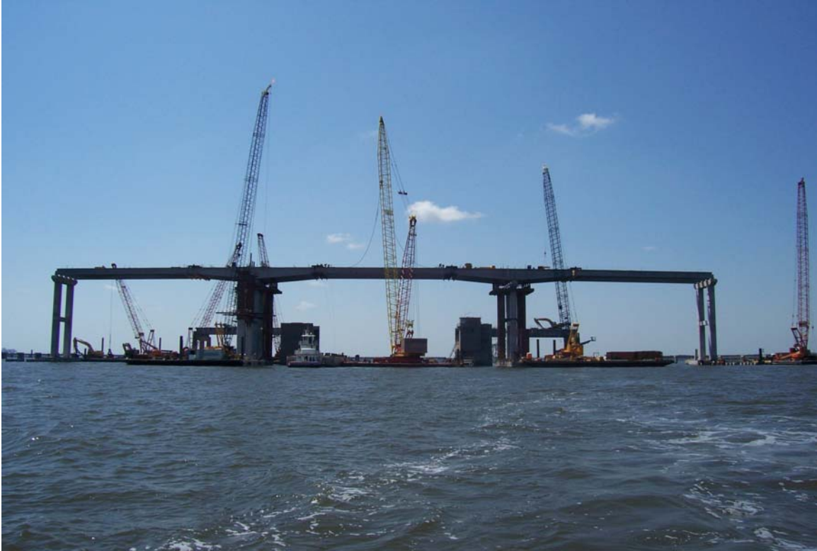
Figure 2 This is U.S. 90 Biloxi Bay Bridge Located in Biloxi, MS
